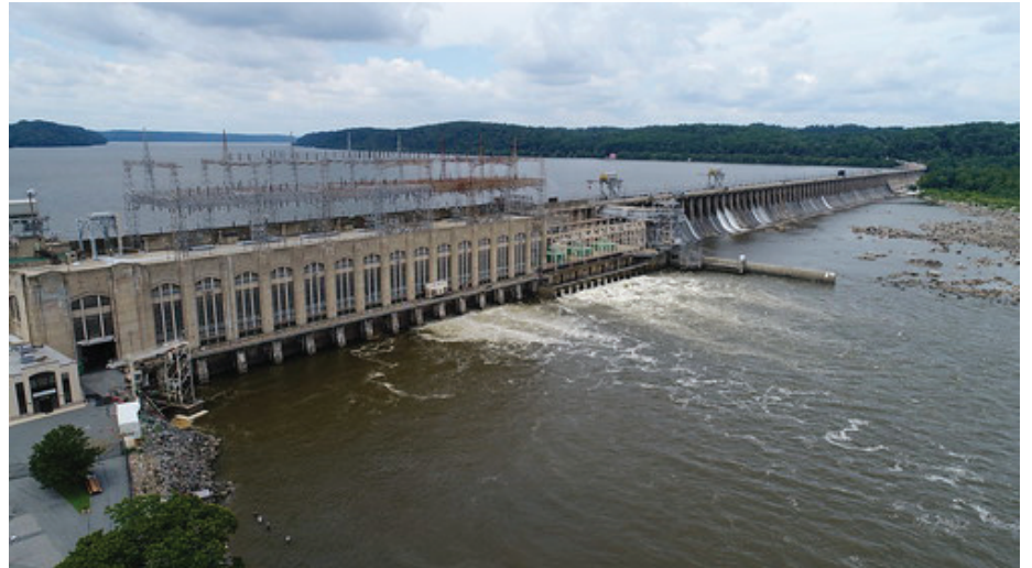
Conowingo Dam stretches across the Susquehanna River between Cecil and Harford counties. Fish lifts built onto the structure help migrating species move upriver, but also catch invasive species. Maryland Department of Natural Resources photo.
